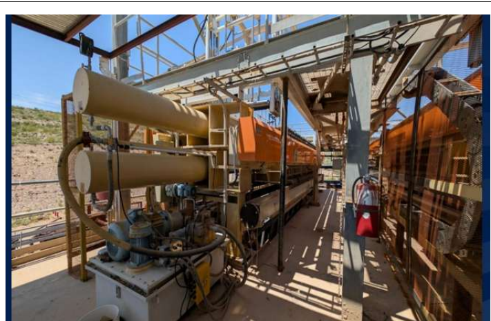
Figure 12: Shafter Processing Facility Filter Press
